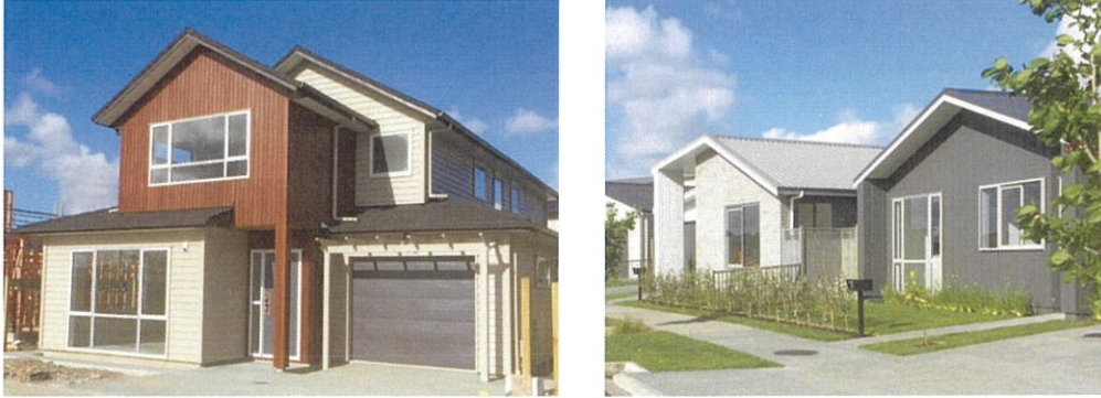
Figure 5: Examples of a variety of roof forms
